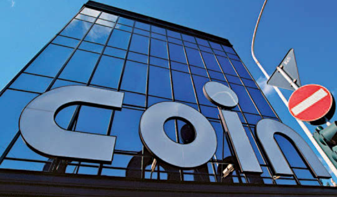
The bold facade of the COIN department store.
